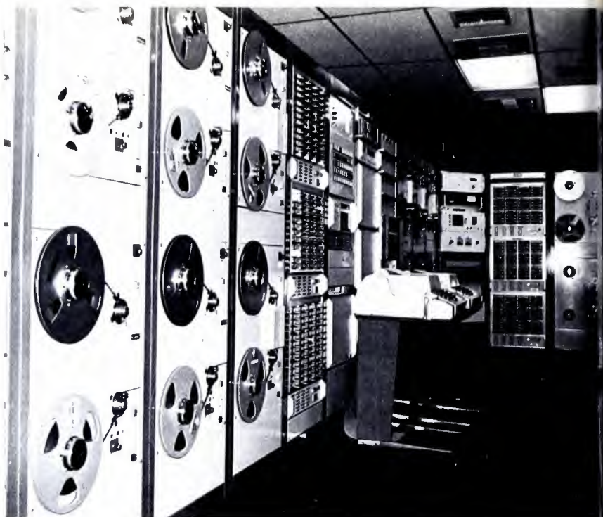
The BT-101 traffic computer generates logs precoded for entering into KBIG/KBRT automation computer (a general automation spec 16). Interface the two systems is part of the Bonneville computer division's long-range plan.
