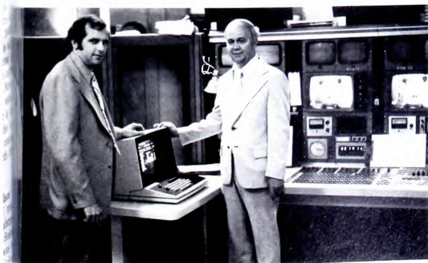
Andy Van Camp (left), engineering liaison, WEWS-TV, and James E. Bloyd, vice president and chief engineer, WEWS-TV, check out master control room of new total automation system.
